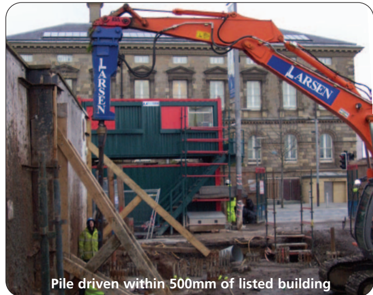
Piling Rig is light weight and handles its own piles
