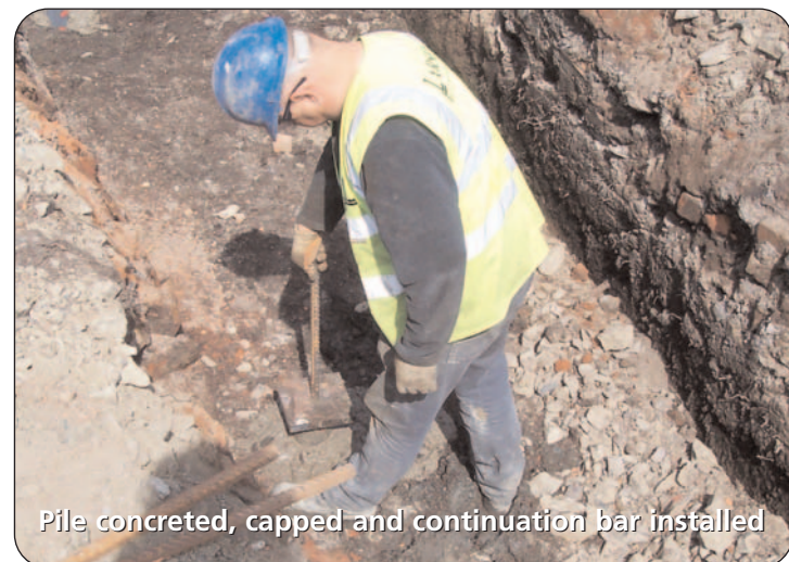
Pile driven within 500mm of listed building
