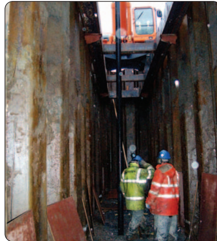
Pipeline inside sheet piled trench
