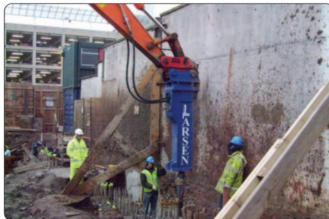
14 Storey building adjacent to a listed building
