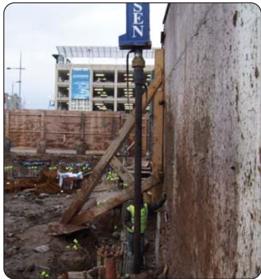
Pile close to listed building
