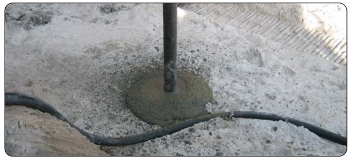
Continuous grouting while pile is driven
