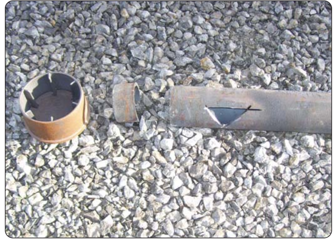
Components for grouted pile
