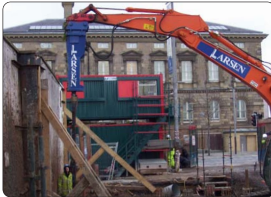
Reach over 4m to pile locations
